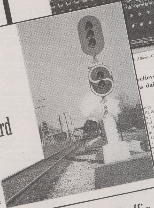
Power switch and signal at a typical end of a siding
