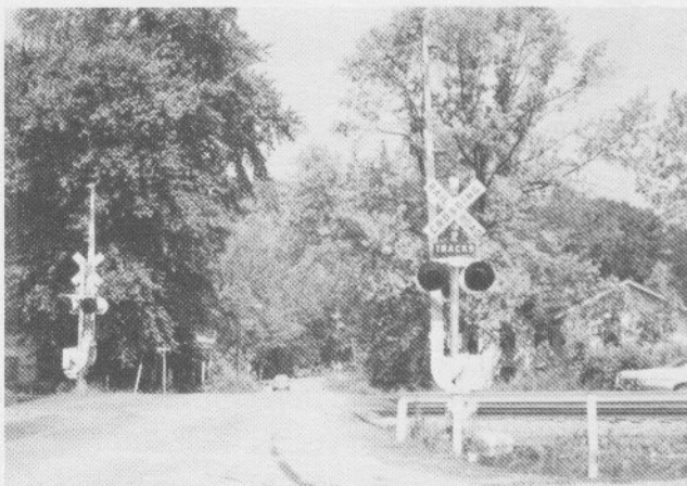
Figure 4- Automatic crossing gates are commonly used adjuncts to flashing-light signals and are required where two or more main tracks cross a highway. In recent years, gates have been installed at single main line crossings where the density of rail or highway traffic warrants the additional safety that gates provide. The gate arms, which are available in wood, fiberglass or aluminum, are raised and lowered by a mechanism containing an electric motor, gears and electrical contacts. Additional lights are mounted on the gate arms. In some cases, a sidewalk arm is used to alert pedestrians.
