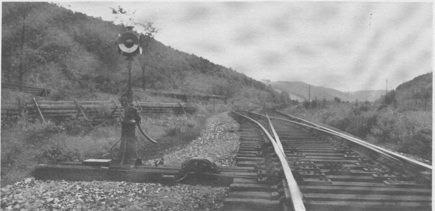
Switch layout with switch circuit controller
